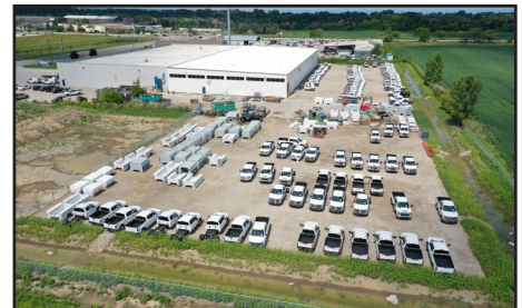
Windsor Manufacturing Facility: 85,000 sq. ft
